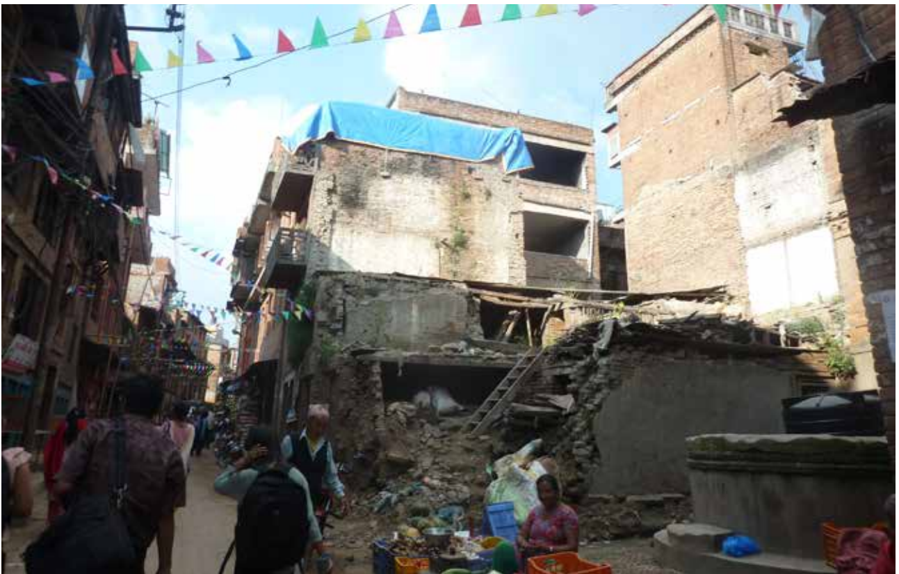
Core area of Bhaktapur. Houses are severely damaged.
